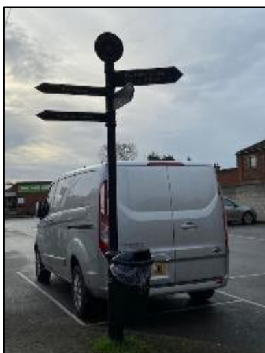
Photo (Southbound): Wayfinding on Chapel Street to station, no distance or walk time indicated and dark sign background makes it difficult to read.
