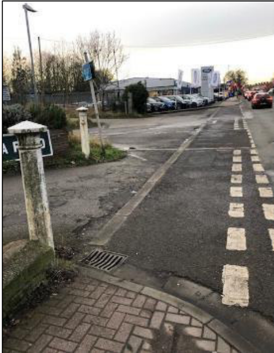
Photo (Left: Northbound; Right: Southbound): excessively wide junction bell mouth and stepped pedestrian access at Summergangs Lane
