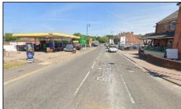
Google Streetview Snip (Eastbound): No pedestrian crossing facilities on the Bridge Road arm
