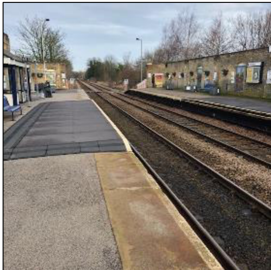
Photo (Northbound): Station platforms with no tactile paving but raised area to improve level access onto trains. Barrow crossing at the far end of the platforms.
