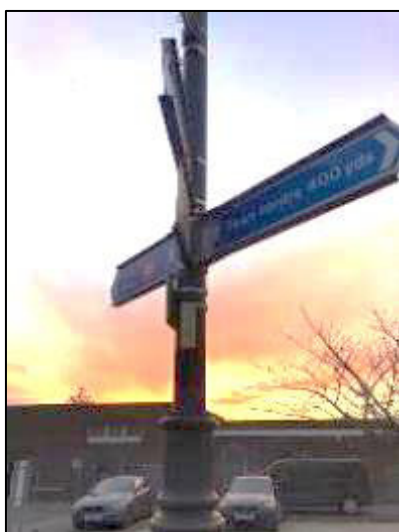
Photo (Westbound): Wayfinding sign opposite Marshall's Yard. Signpost not correctly orientated
