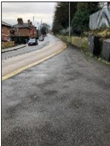
Photo (Southbound): Station Road wide footway with potential for on/off-slip cycle lane to Harlaxton Road.
