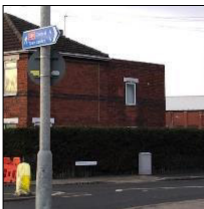
Photo (Northbound): Wayfinding signage at Ashcroft Rd/Lea Rd roundabout. Signpost not correctly orientated
