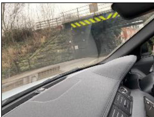
Photo (Southbound): Poor visibility from Station Approach to Ermine Street, footway on opposite side of the road.
