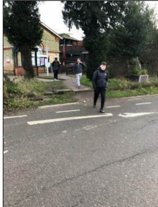
Photo (Left: Northbound; Right: Southbound): excessively wide junction bell mouth and stepped pedestrian access at Summergangs Lane
